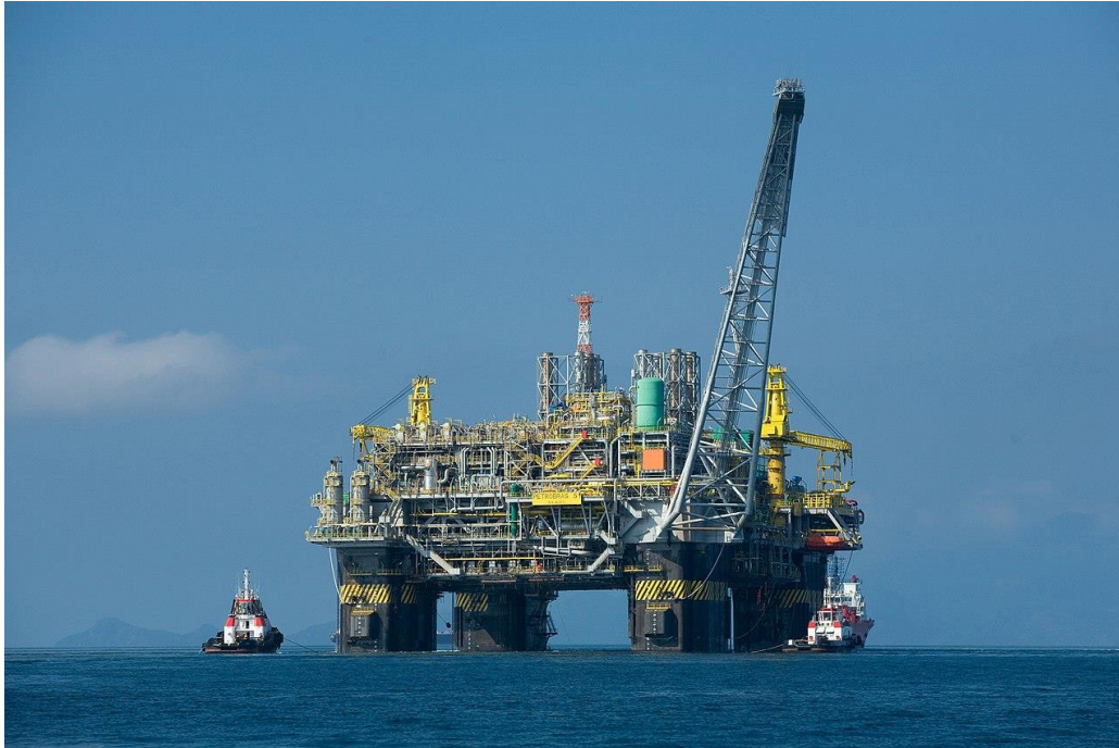
Oil platform P-51 off the Brazilian coast is a semi-submersible platform. Divulgação Petrobras / ABr - Agência Brasil [1]
