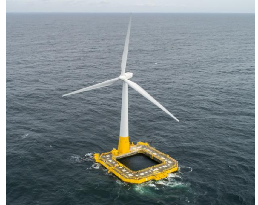
The Floatgen floating wind turbine, equipped with the Ideal float, installed on the SEM-REV (Centrale Nantes) off Le Croisic. Credits: Ideol / V. Joncheray
